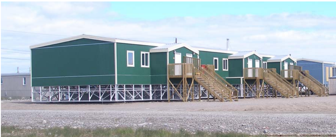
Figure 1: Completed NHC 5-Plex in Arviat, Nunavut
