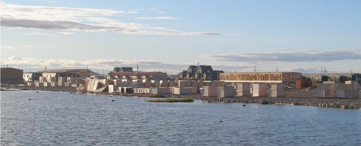
Figure 3: Sea Lift Materials and a 5-Plex's Under Construction in Arviat
