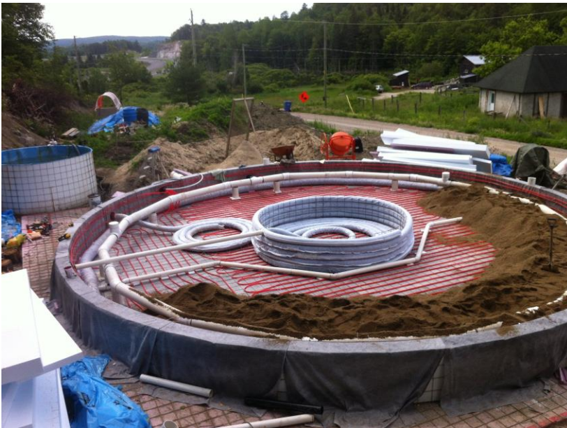
Foundation Thermal Storage Battery Lagoon and Digester.
